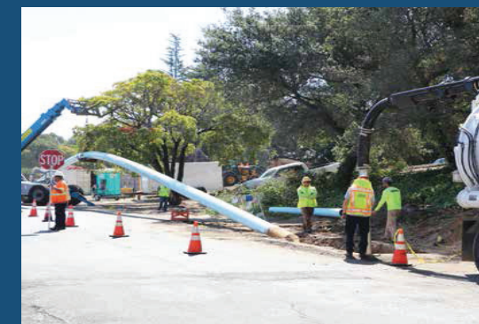
Beginning pipeline pullback on Old Sonoma Road.
