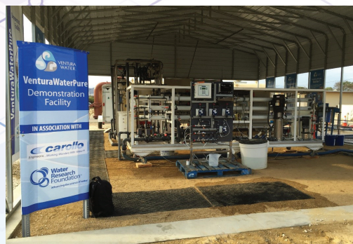
Demonstrating continuous 4-log removal of a fluorescent molecular marker (Trasar) through RO membranes in Ventura, CA, takes a big bite out of total disinfection requirements for potable reuse!
