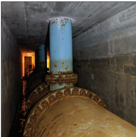
Figure 1. Discharge header pipe tunnel.
