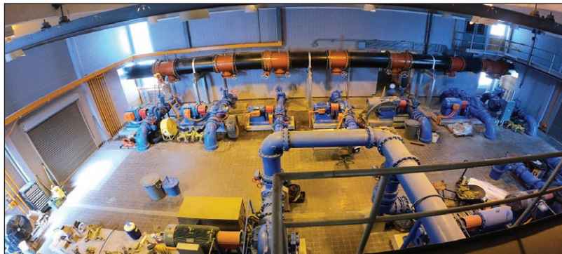
Figure 13. Phase 2 – Header pipe construction.
