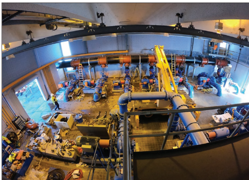
Figure 14. Phase 3 – Tie-in of pumps to header.
