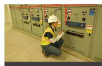
Extensive additions to the power infrastructure including 15kV, 5kV, and 480V SWGR, and 480V MCC's, all featuring a digital bus for communications.
