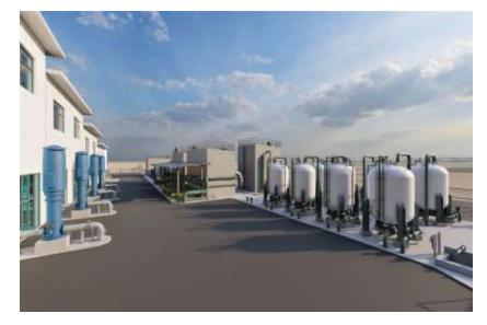
The facility will have a redundant treatment train that includes multiple polishing steps, including advanced oxidation and granular activated carbon.
