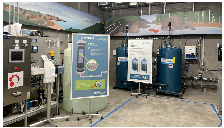
Steps 2 and 3 of the Pure SoJo treatment train are ultrafiltration and granular activated carbon.
