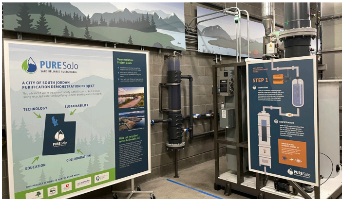
Step 1 of the Pure SoJo treatment train is ozone and biologically active filtration, or biofiltration.
