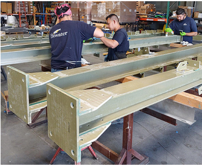
FRP membrane supports being fabricated in Bewater's shop
