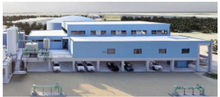
FKAA's Hurricane-proof SWRO crib
